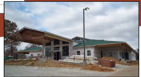
PINNACLE MONTESSORI SCHOOL CURRENT CONSTRUCTION
